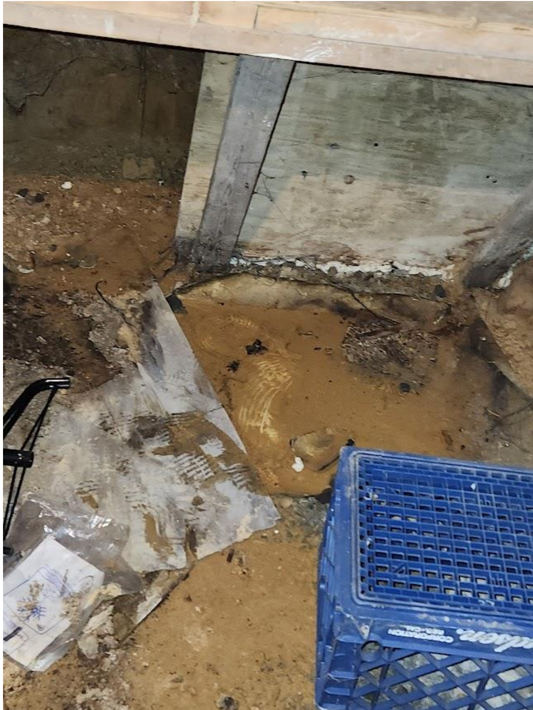
Photo 2: Water Intrusion in Basement
