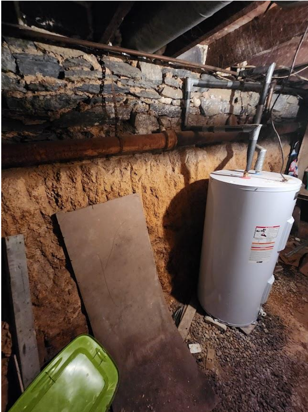
Photo 1: Dugout Portion of Basement with Stacked Stone and Dirt Walls
